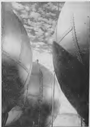
When Gulliver got lost in the land of the Broodingtops, he happened across a sports field and climbed up on one of the footballs. This is probably how it looked. Or getting back to earth, this is an employer inspecting Laga's big silver gas spheres.
